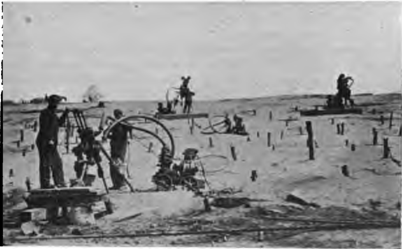
PLATE 184b. —Contract 9. Quarry and Temple-Ingersoll Electric Air Drills at Work. Pulsator for drill in foreground.
